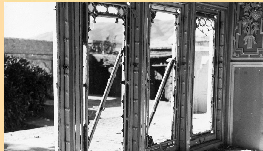
Interior of the historic 19th century home of the Báb after its 1979 destruction (Credit: Bahá'í International Community)
